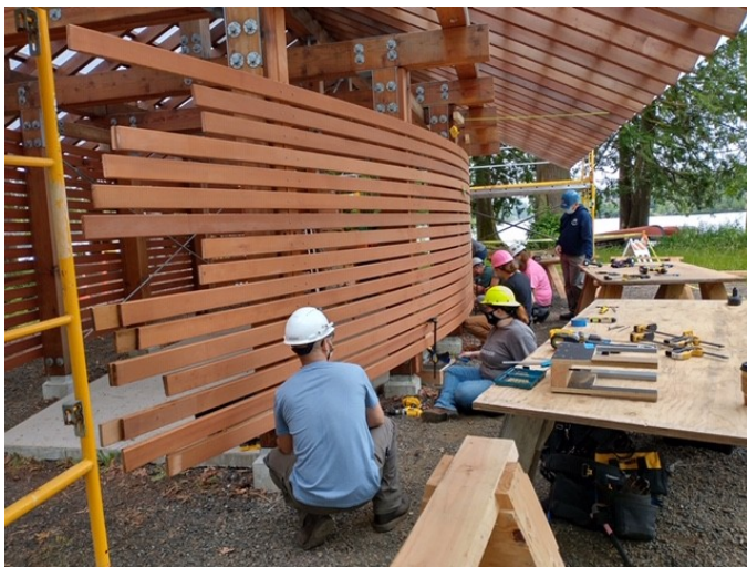
Laminated cedar siding planks installed on building: 2020
