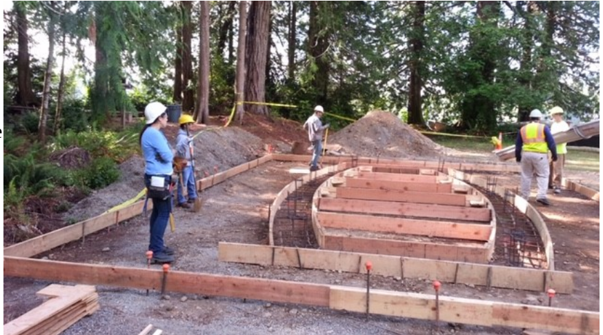
Site preparation and form building for the Canoe House pad: 2016
