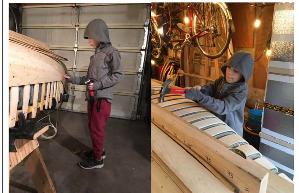
Matthew nailing planks.
